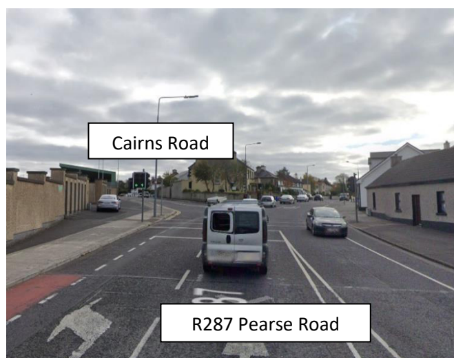
Plate 2 – R287 Pearse Road / Cairns Road Junction
