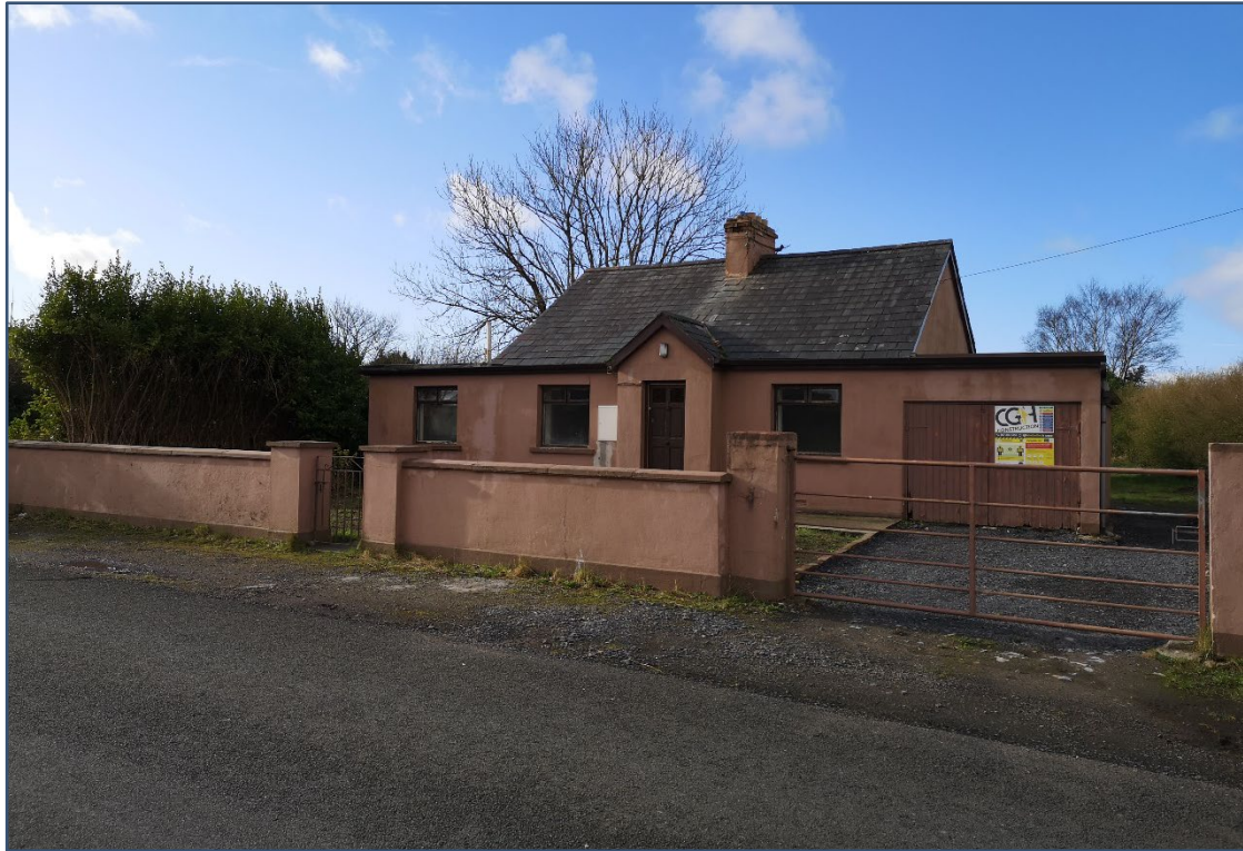
Plate 3-7 Derelict building in the northeast corner of the site
