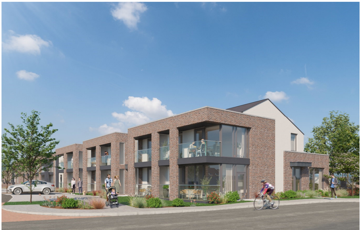
3-D Visualisation of typical Apartment/ Duplex Block showing Brick, Render & Glazed Materials to facades with tile pitched roofs over
