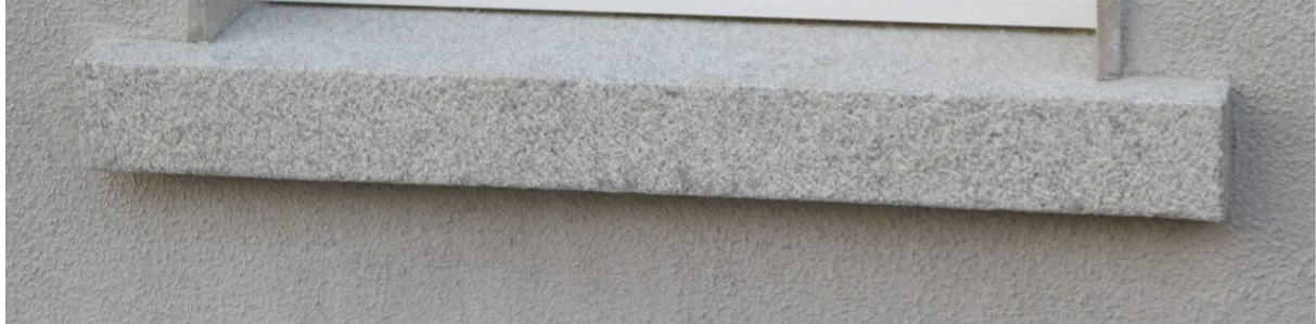
Image of RC Window Cill/ Parapet type
