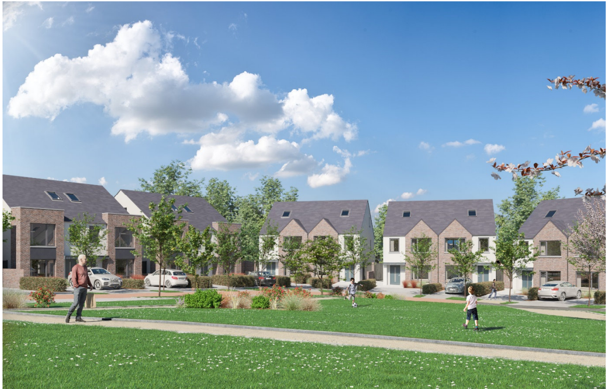
3-D Visualisation showing typical House Blocks showing Brick, Render and Pressed Metal Materials in differing compositions to facades with tile pitched roofs over
