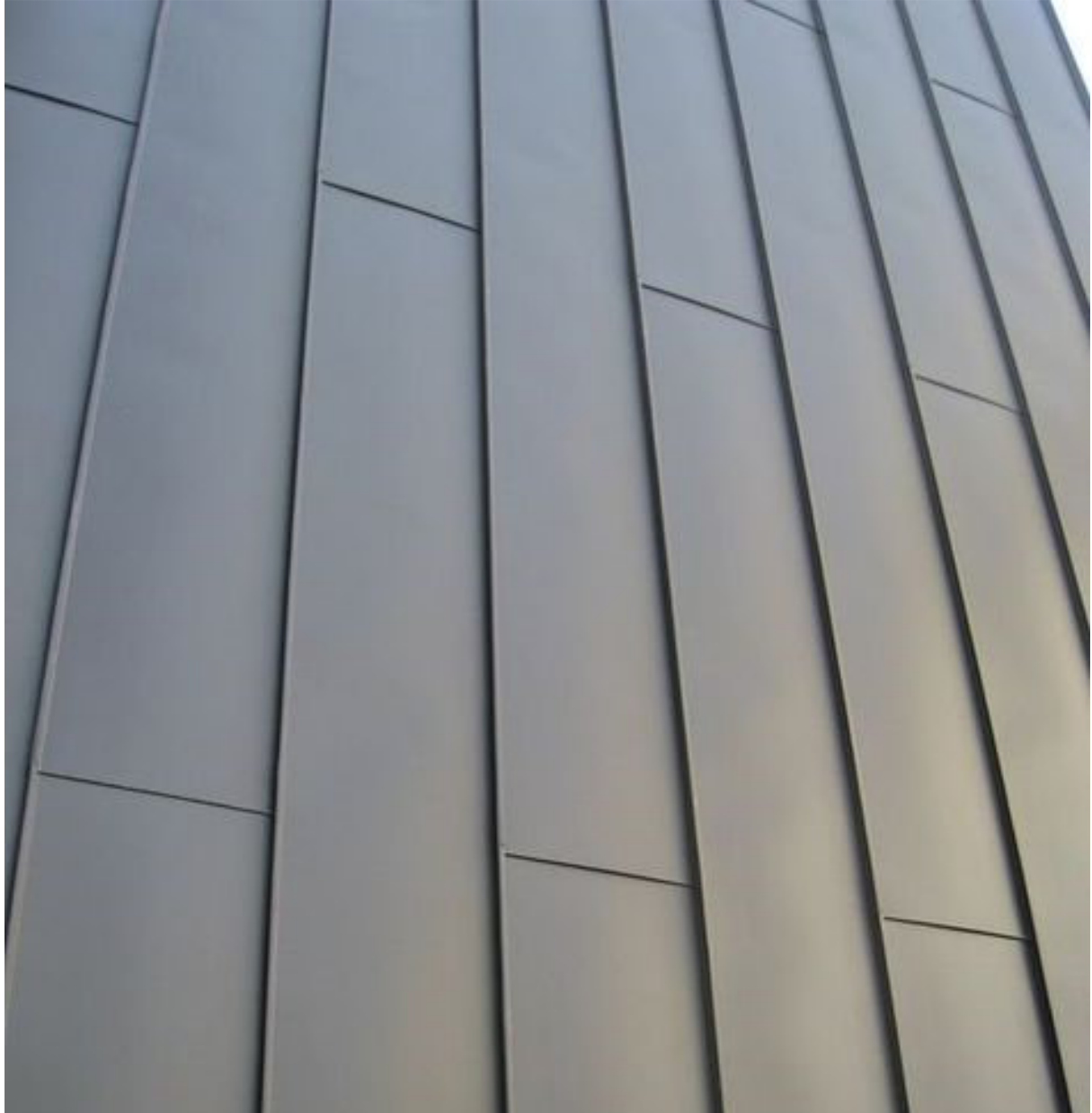
Dark Grey Coloured Pressed Metal Cladding to Canopies at Unit Entrances
