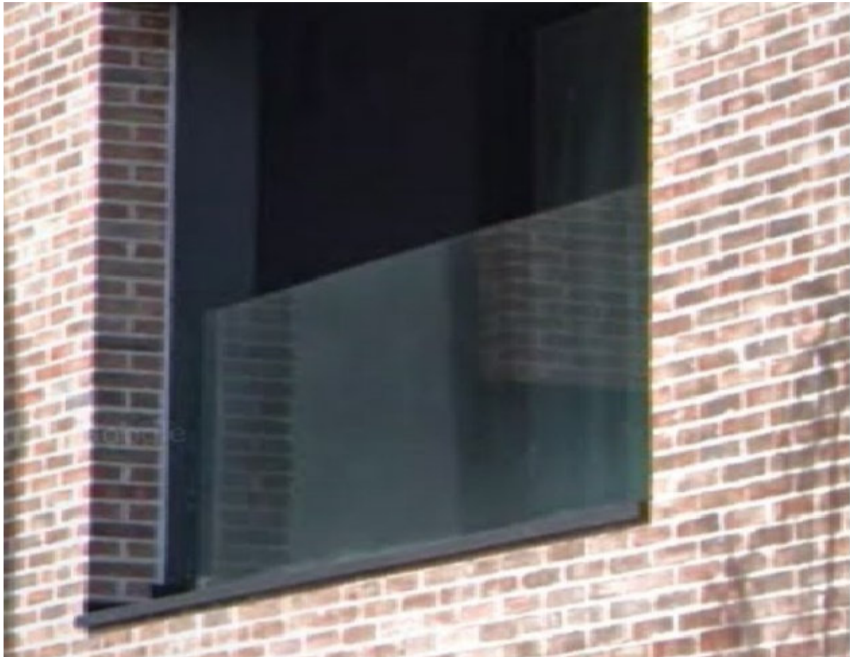
Image of Glazed Balustrades to External Terraces
